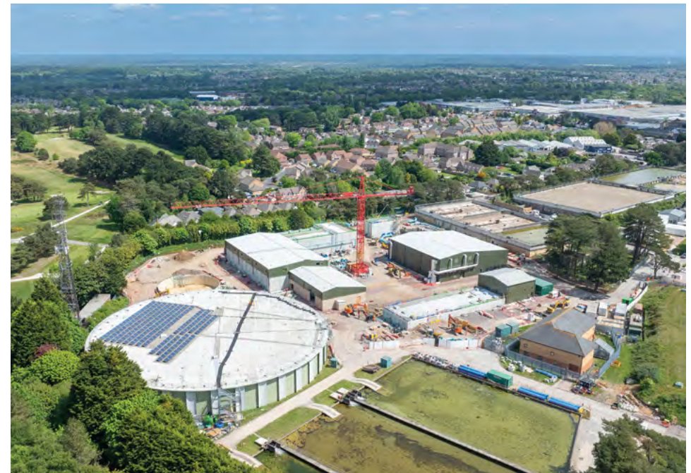
Alderney build in progress
