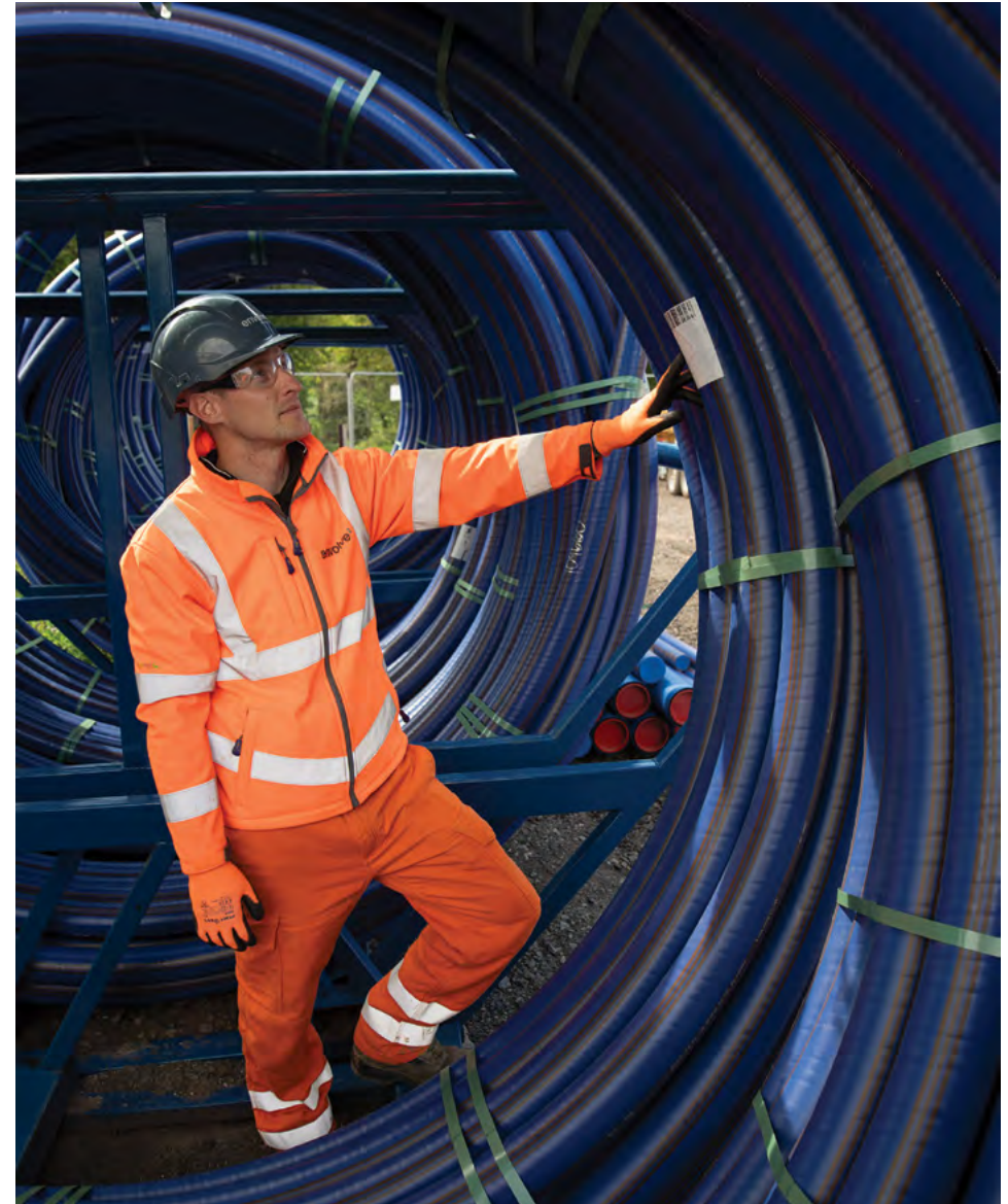
④ Bristol mains repairs
