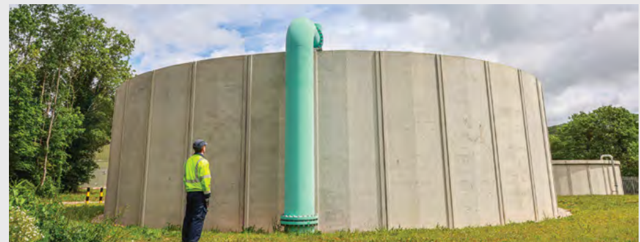
Littlehempston Water treatment works
