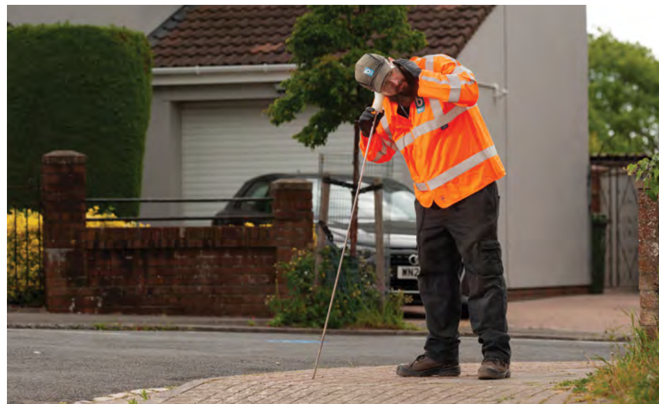
Leakage detection in Bristol
