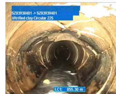
Collapsed pipe
