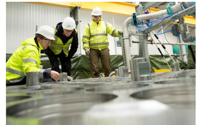
Ceramic SIX® filters, Mayflower Water Treatment Works
