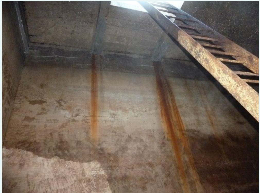
Alderney Service Reservoir
