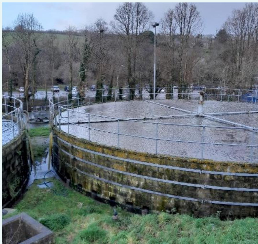
Helston Wastewater Treatment Works
