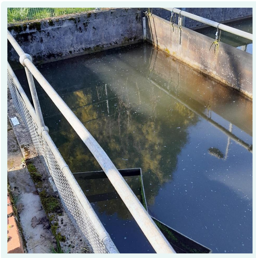
Stowey Water Treatment Works
