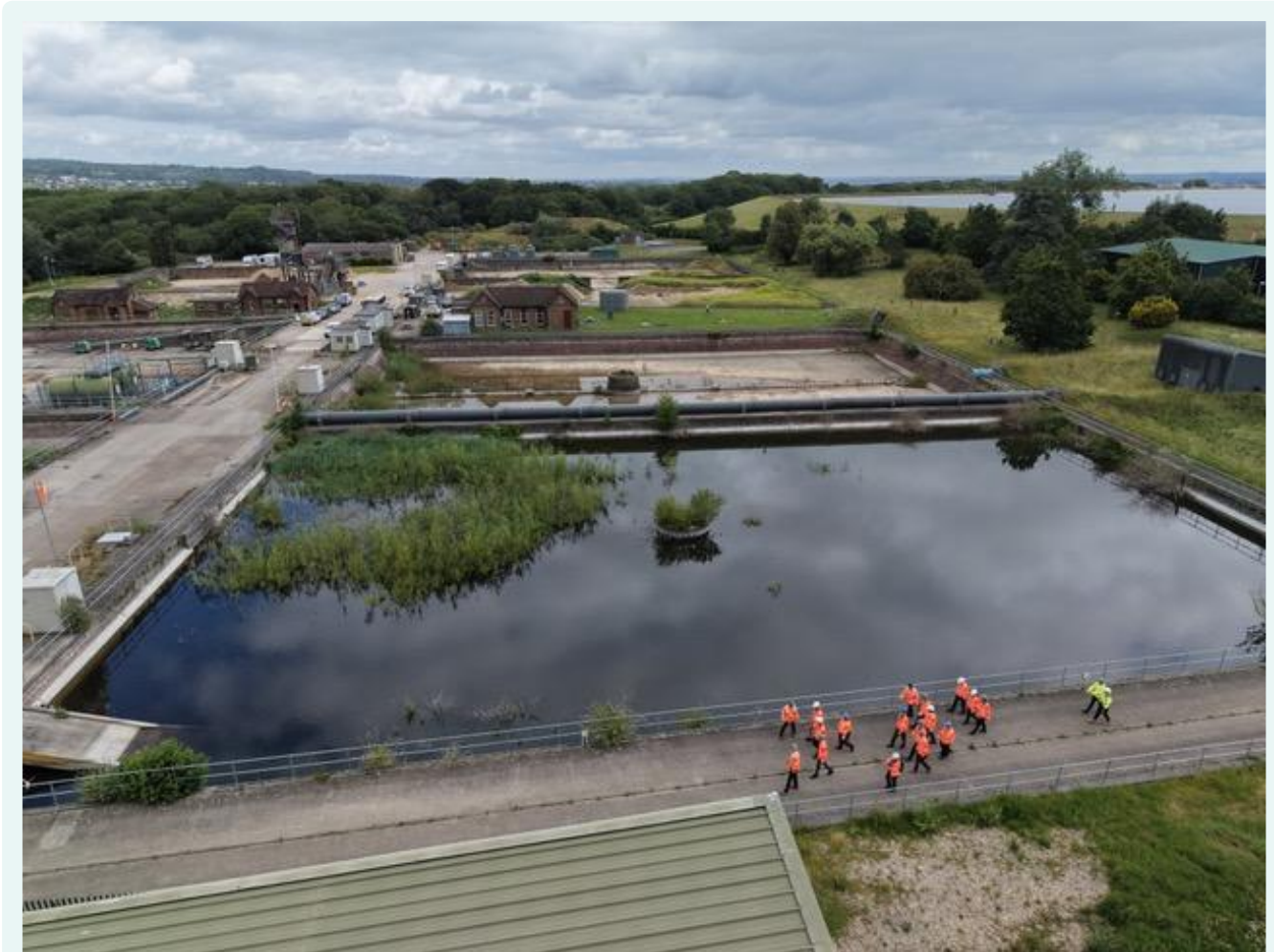
Barrow Water Treatment Works
