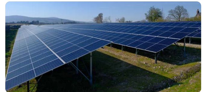
From top to bottom Storm tank construction at Dawlish, Devon; Alderney Water Treatment Works, Bournemouth; solar panels at Cullerlie, Scotland
