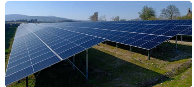
From top to bottom Storm tank construction at Dawlish, Devon; Alderney Water Treatment Works, Bournemouth; solar panels at Cullerlie, Scotland
