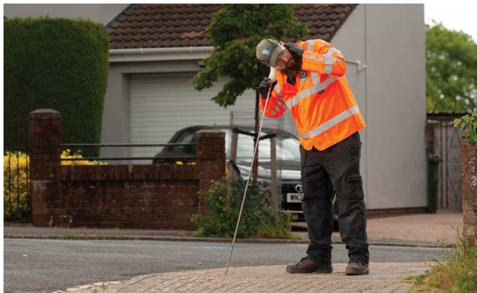
Leakage detection in Bristol
