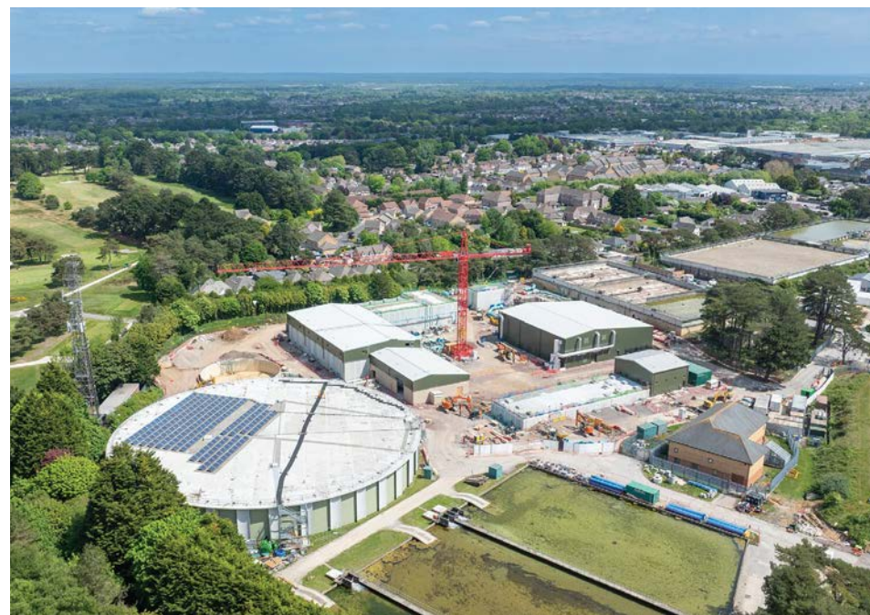
Alderney build in progress
